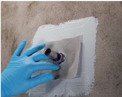
Application of a Mapeband PE 120 seal for through holes using Mapegum WPS
