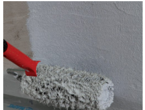
Application of Mapegum WPS with a roller
