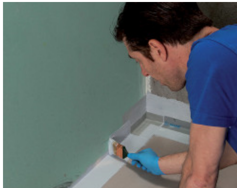
Application of Mapeband PE 120 using Mapegum WPS
