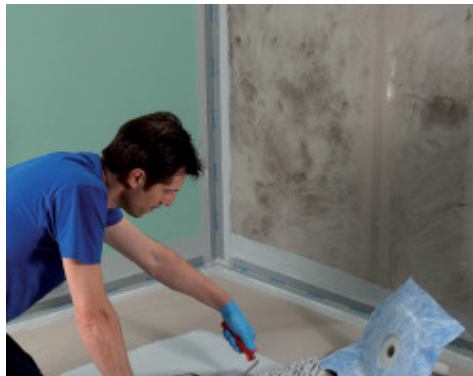
Application of a Drain Vertical fitting using Mapegum WPS
