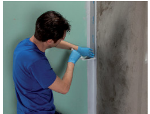
Application of Mapeband PE 120 using Mapegum WPS
